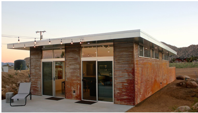
Yard Building - Cottage Home
