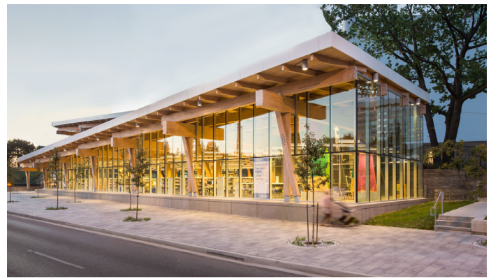
Civic Building - Library
