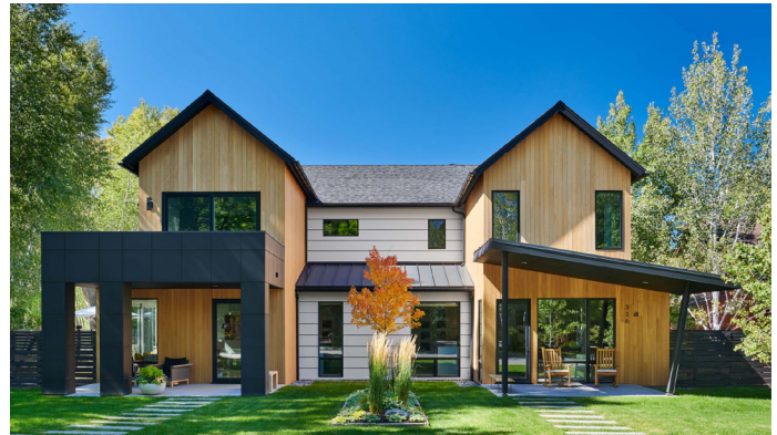
Yard Building - Duplex
