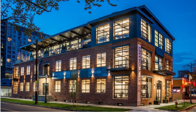
Storefront Building - Office
