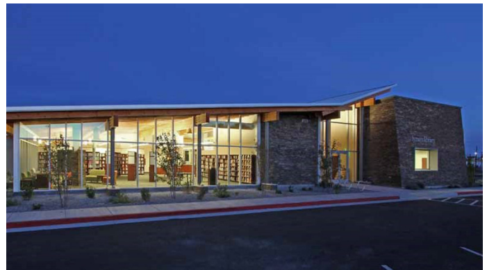
Civic Building - Small-scale Library
