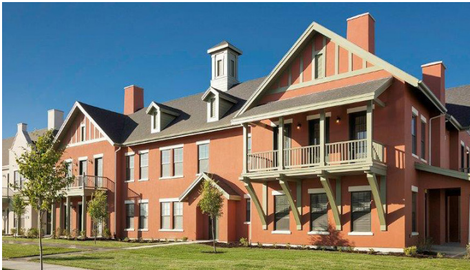
Yard Building - Mansion Apartments
