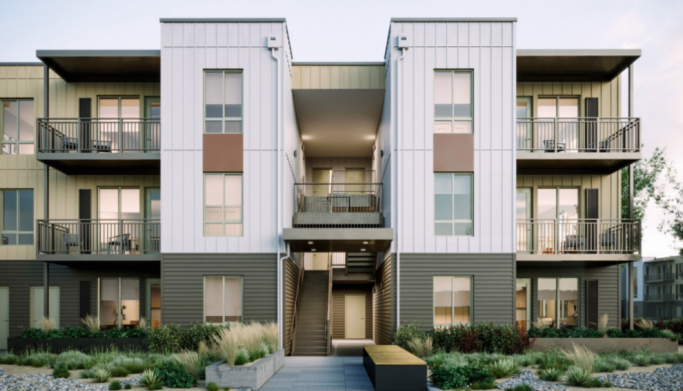
Stoop Buildings - Multiplex
